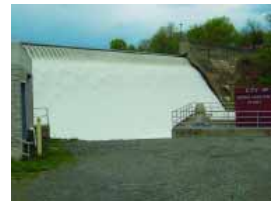
Our fiber optic capabilities provide City of Manassas employees with remote access to their water treatment plant.
