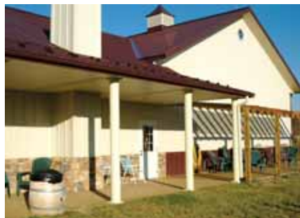
Pearmund Cellars winery, tasting room and retail store use smart architecture and geothermal energy for maximum heating and cooling efficiency.
