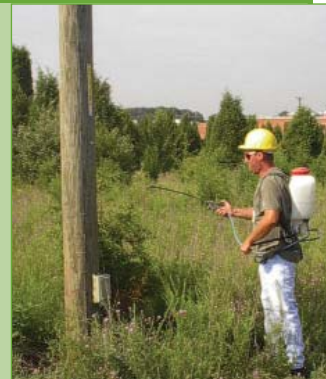
Backpack sprayers are used to apply herbicides to targeted areas within NOVEC rights of way.
