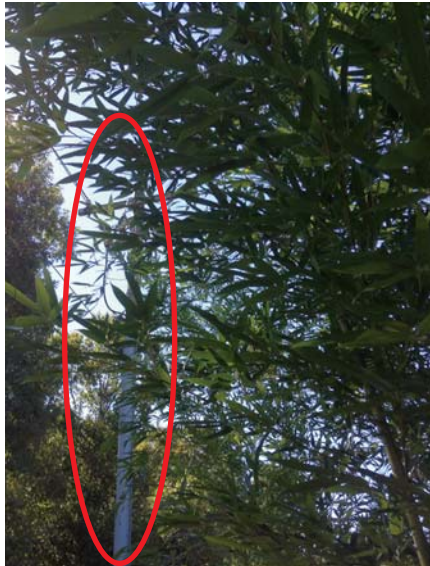
Overgrown bamboo that conceals a power line creates a potentially dangerous situation.
